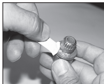
Apply Lubricant to Hub
